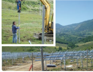
Tornillo de tierra Ground screw
