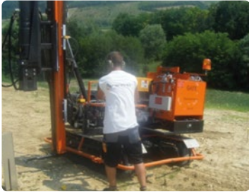
Hincado directo Pile driving
